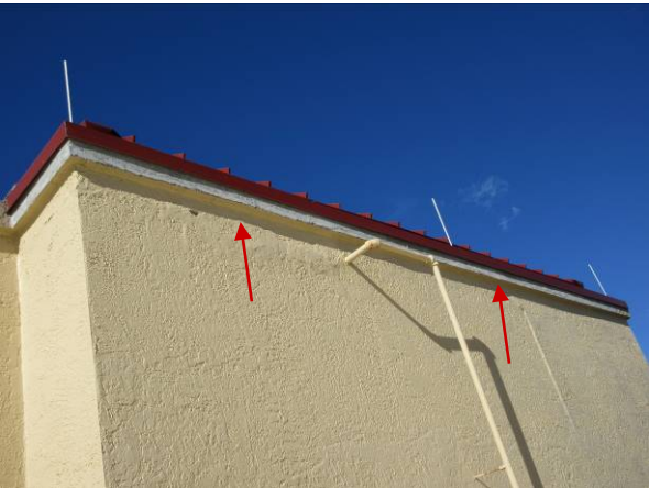
Photo #28 – Roof – typical unpainted stucco repair.
