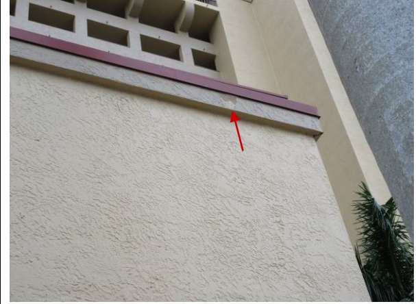
Photo #64 – Front of tower – blister in paint on pillar.
