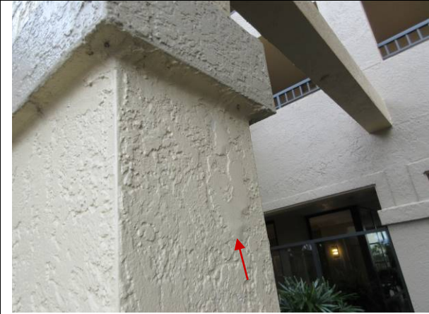
Photo #64 – Front of tower – blister in paint on pillar.
