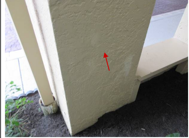
Photo #63 – Front of tower – peeling paint on pillar.
