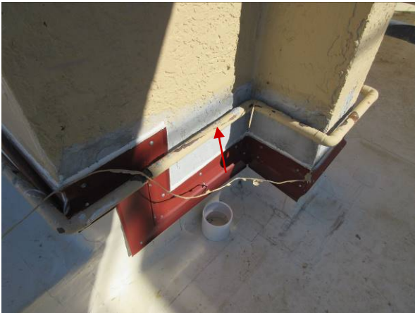
Photo #27 – Roof – typical unpainted stucco repair.
