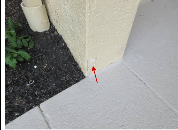
Photo #63 – Front of tower – peeling paint on pillar.
