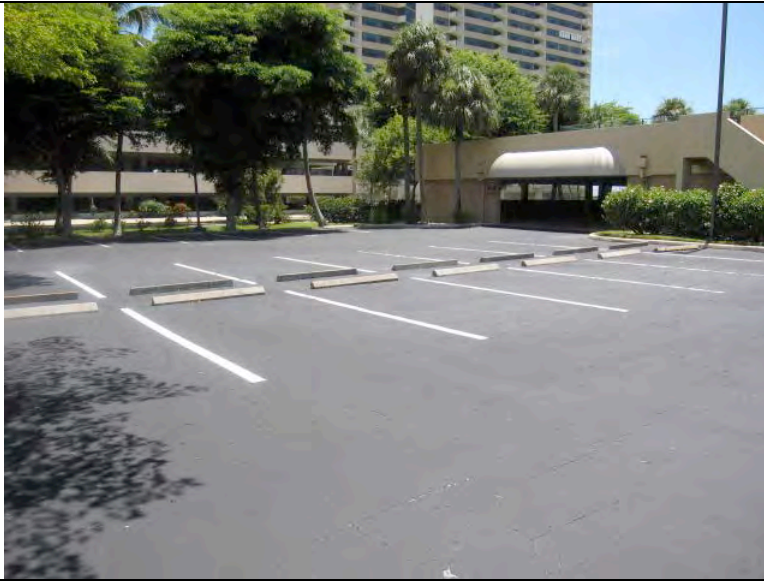
Paving, Asphalt Sealcoat & Restripe
