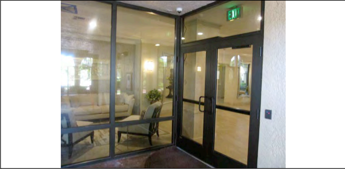
Front Entry Doors and Jambs
