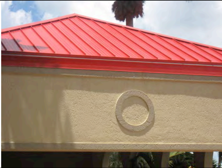
Painting, Portico Roof
