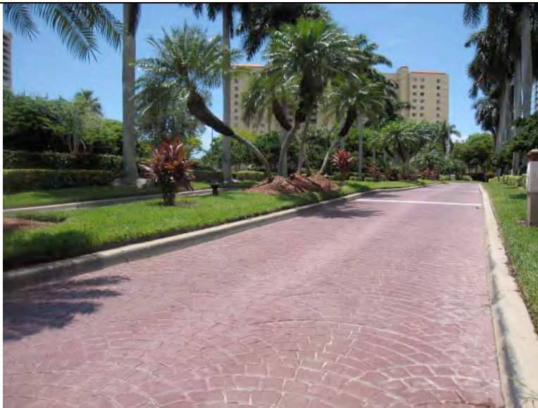
Paving, Bomanite Reseal
