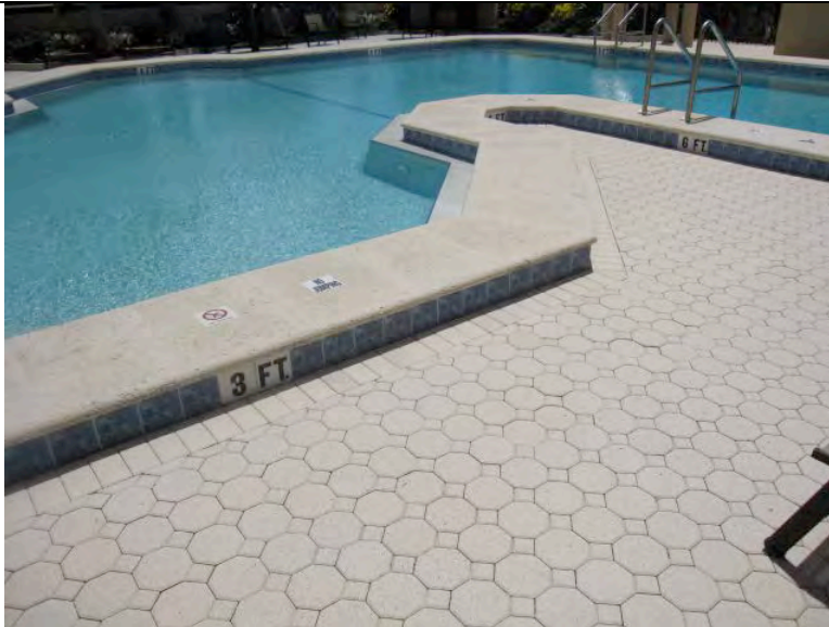
Pool Deck Pavers
