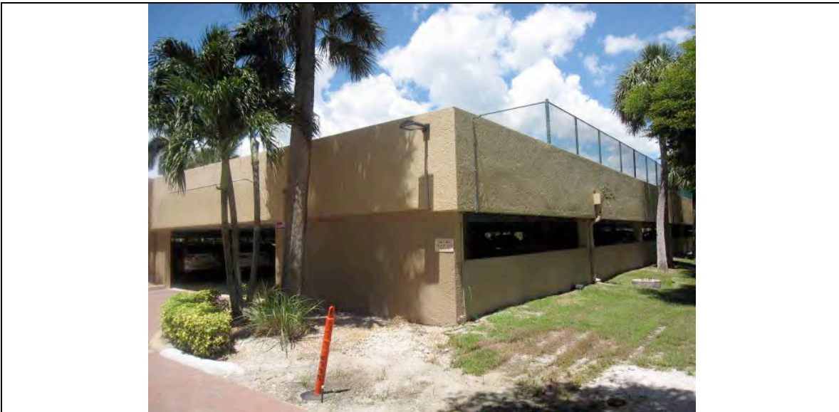
Roofing, South Garage
