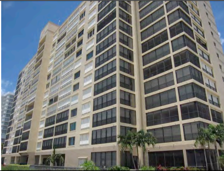
Screened Balconies & Railing
