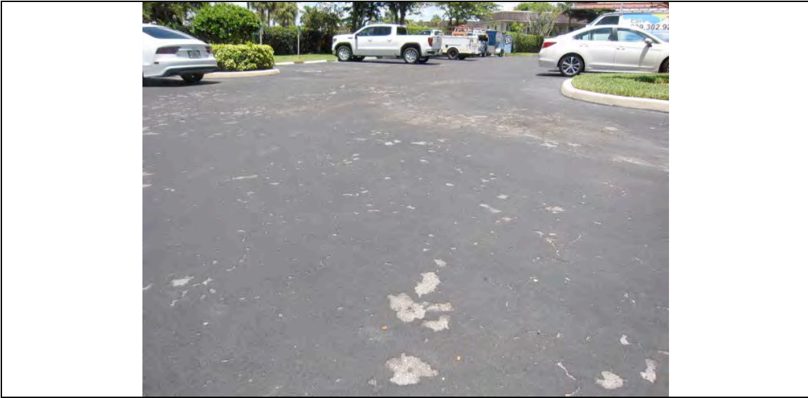
Paving, Asphalt Overlay
