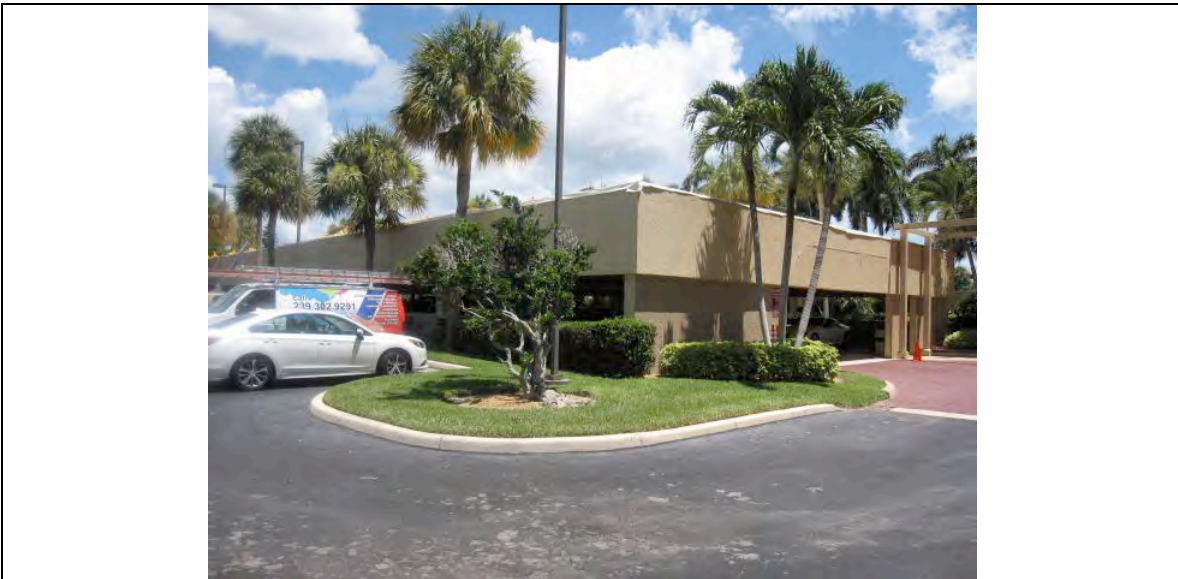
Roofing, North Garage
