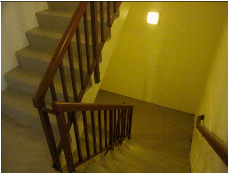
Stairwells & Railing, Repaint
