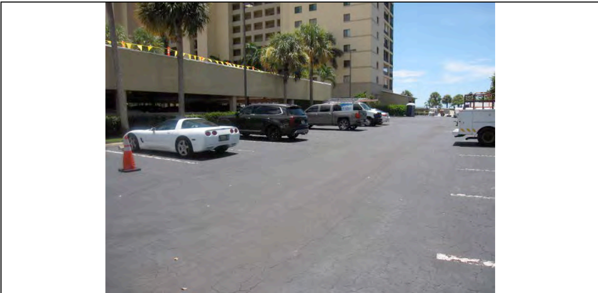
Paving, Asphalt Overlay
