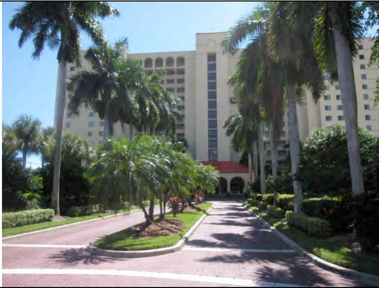
Painting, Exterior, Tower
