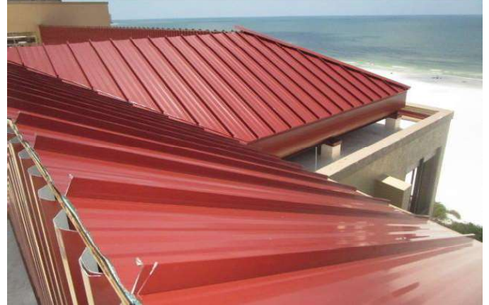
#2) roof covering: 2021 METAL mansards w/2021 duro-loc type flat vinyl roof #ROOF-20-02858 3/16/2021
