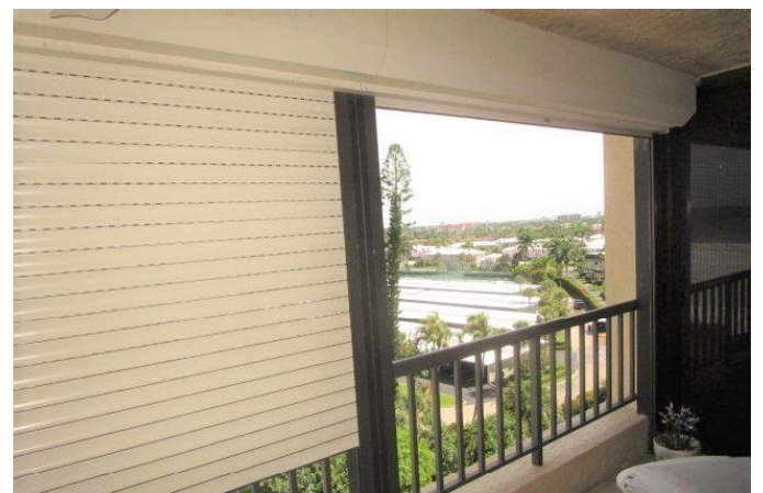
#7) opening protection: non impact rear sliders w/roll down shutters #WD-17-05424 applied 7/28/2017
