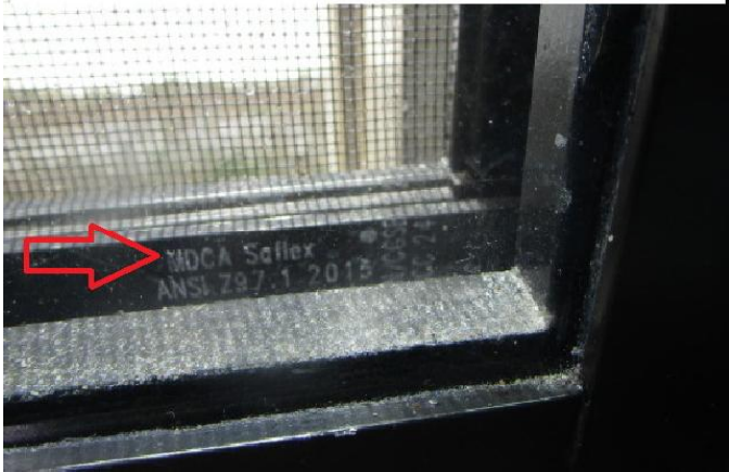
#7) opening protection: impact rated window mfg watermark MDCA=mia-dade county approved
