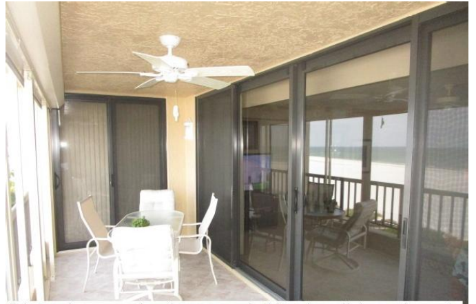
#7) opening protection: impact rated sliders (& roll down shutters) permit WD-17-09469 applied 12/14/2017
